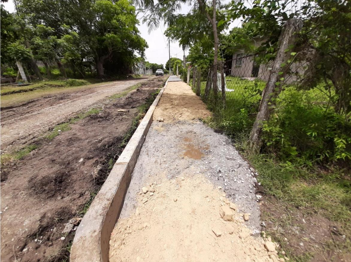
0035 RELLENO EN ZANJAS CON MATERIAL INERTE EN CAPAS DE 20 CMS. DE ESPESOR POR MEDIOS MECANICOS AL 90% PROCTOR.
